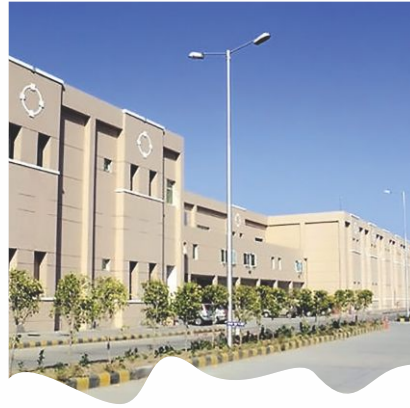
Patanjali Industrial Park
